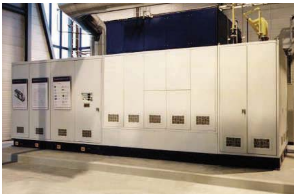
Pure and simple. Solid-oxide fuel cells, such as the ones in this 100-kilowatt heating plant in the Netherlands, require sulfur-free hydrogen.
